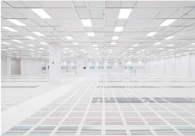
26,527 SF main cleanroom operating at class 100
