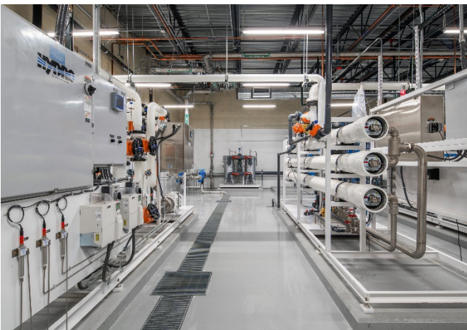
Water processing equipment
