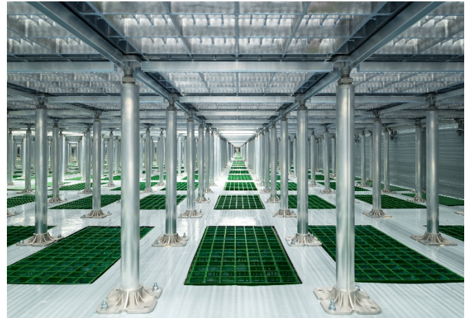
Crawl space between cleanroom and sub fab
